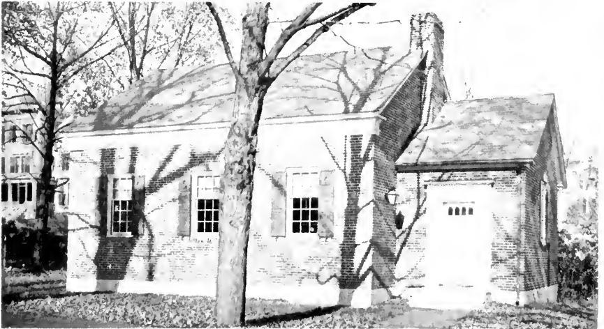
FRANKFORT, KY., LONG LINES REPEATER STATION HARRY HAKE & HARRY HAKE, JR., Architects
